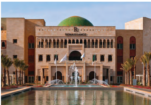
RENAISSANCE TLEMCEEN MARRIOT HOTEL Tlemcen, Algeria 2014
